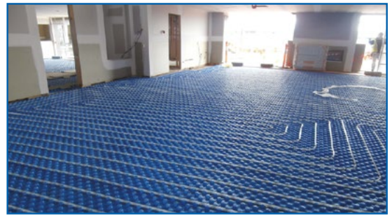
▲ Emmeti floor panels with Emmeti Gerpex Multi Layer 16mm pipe
