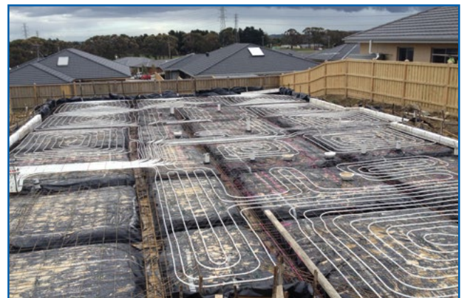
▲ Emmeti PE-Xa in slab application, attached directly to the slab reinforcement
