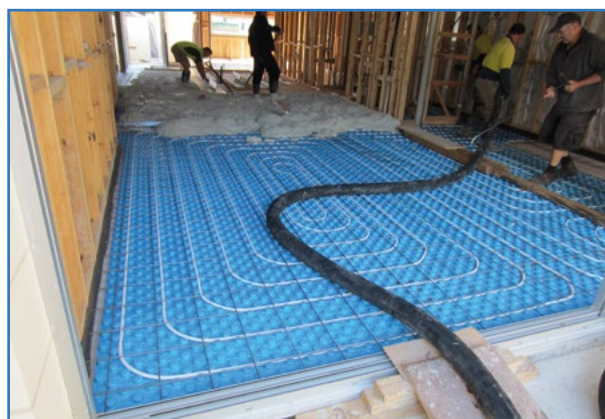
Gerpex Multi Layer pipe with Emmeti floor insulation panels in Screed application
